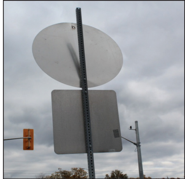
New, no heavy truck sign. The top fastener on the “new” sign has failed. Planning is required to determine whether the sign fasteners should be replaced or if the “new” portion of the sign can be removed.
